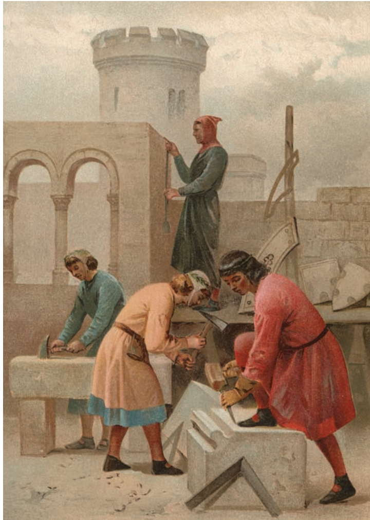
Freemasons at work in the tenth century
